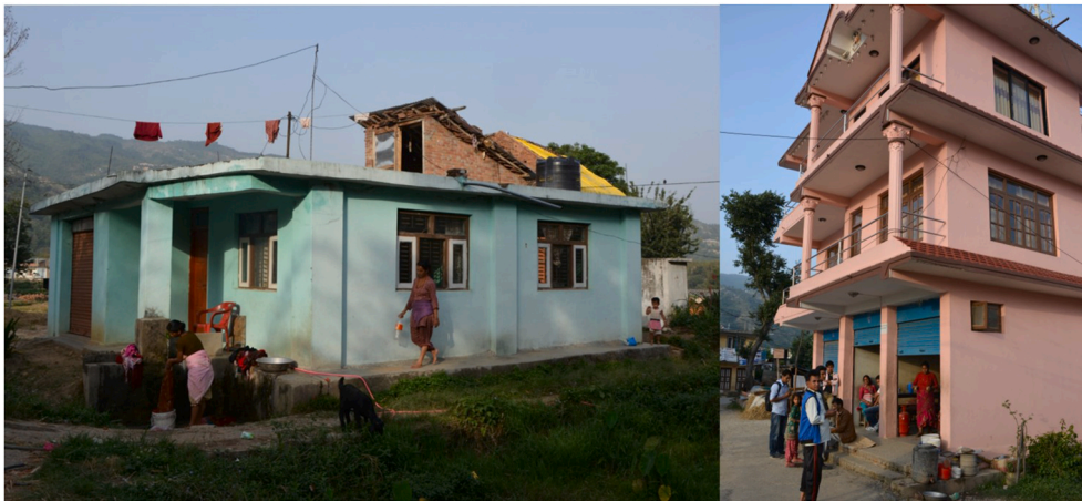
Fig. 8. The retrofitted houses in Aalapot sustained no damage. (Left: newly constructed house based on the advice, right: Student C's retrofitted house).
